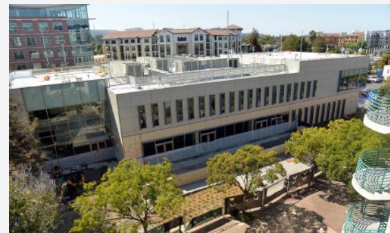
Work on the County's new Regional Operations Center, or ROC, was substantially completed during the 2018-19 fiscal year. The 37,000-square-foot ROC will become the County's hub for disaster planning, response and recovery.
